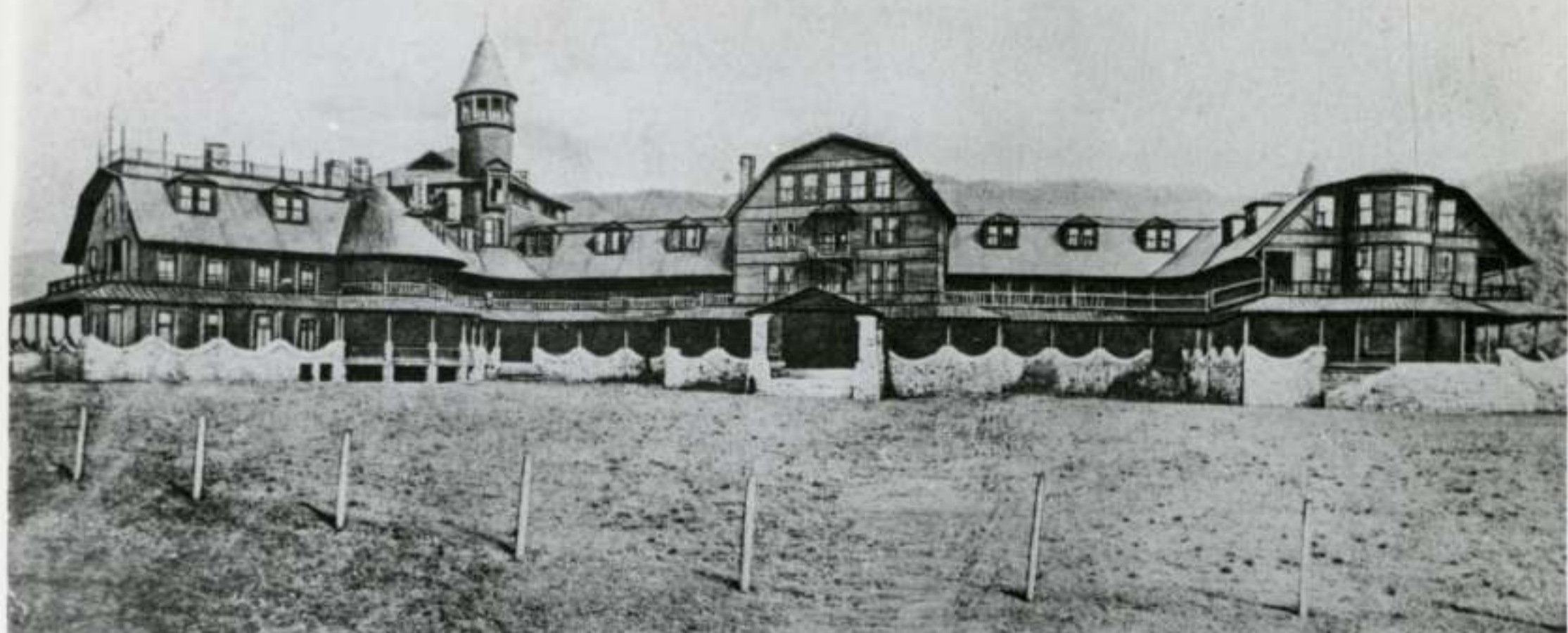
Rockbridge Hotel, Glasgow, Va. Walter H. Robertson & S. R. Leckey-Owners.
