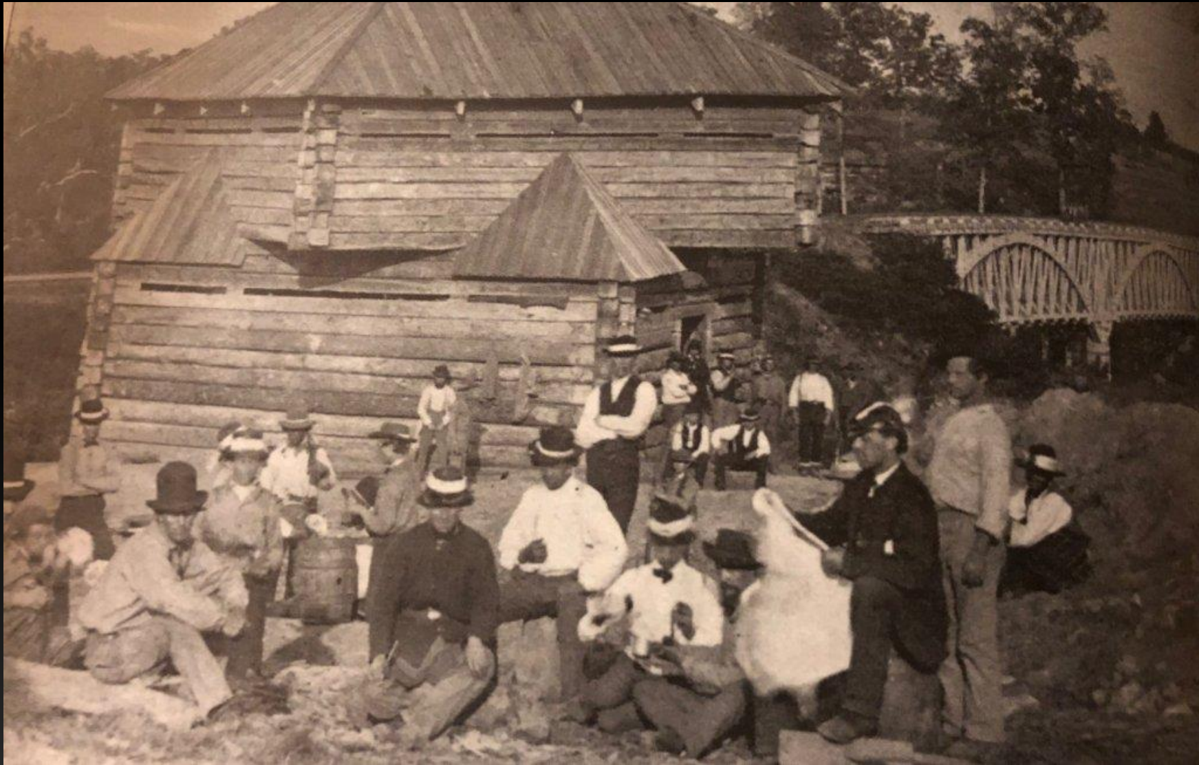
Feb. 1863: Archer Alexander warns Krekel's Deutsch (Union Home Guard) He overhears & foils a pro-Confederate plot to destroy Peruque Bridge (above) Timbers sawn through, to collapse under the next Union train
