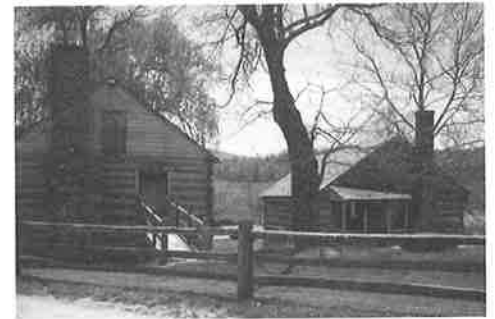
Front view of Blacksmith Shop and Mill
