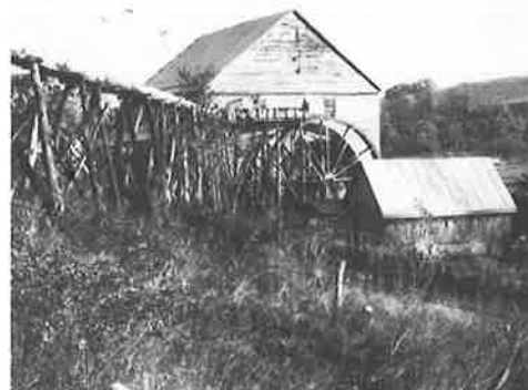
Beatty's Mill showing mill race taken while wheel was running 17 October 1939
