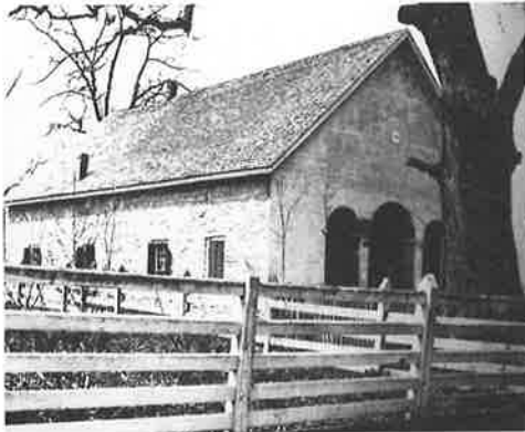
Timber Ridge Presbyterian Church
