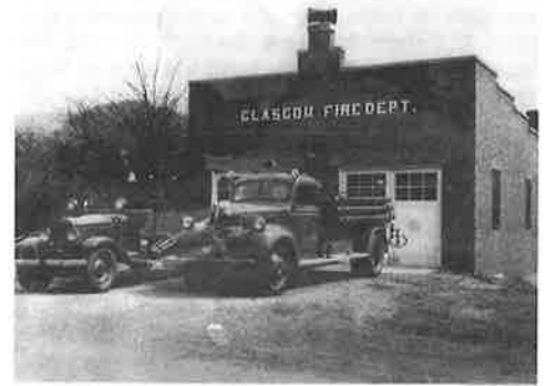
Old Firehouse, with original trucks
