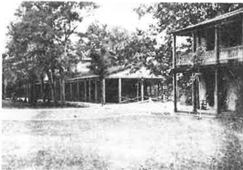
Liberty Hall and Tennis Court
