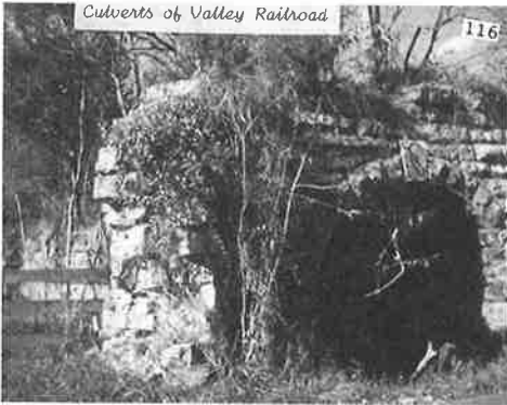
Valley Railroad Culvert on Plank Road
