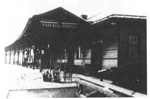
Natural Bridge Train Station.
