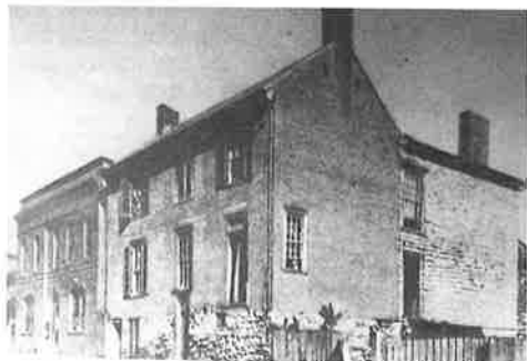
Jackson House before restoration
