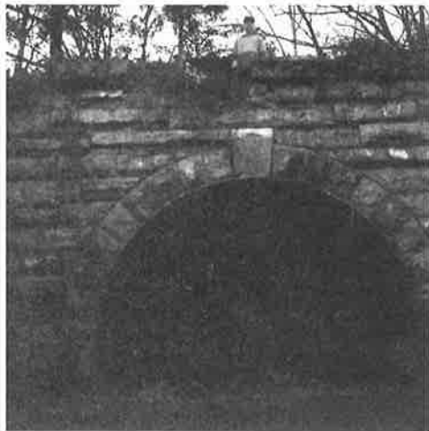
Stone Culvert on Plank Road, remnant of Railroad.
