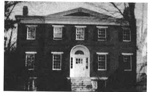
Rockbridge County Jail in Lexington, VA
