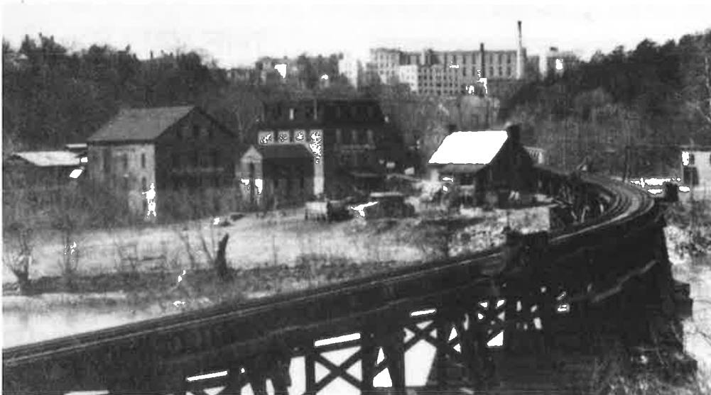
East Lexington, railroad trestle crossing Maury River, 1937
