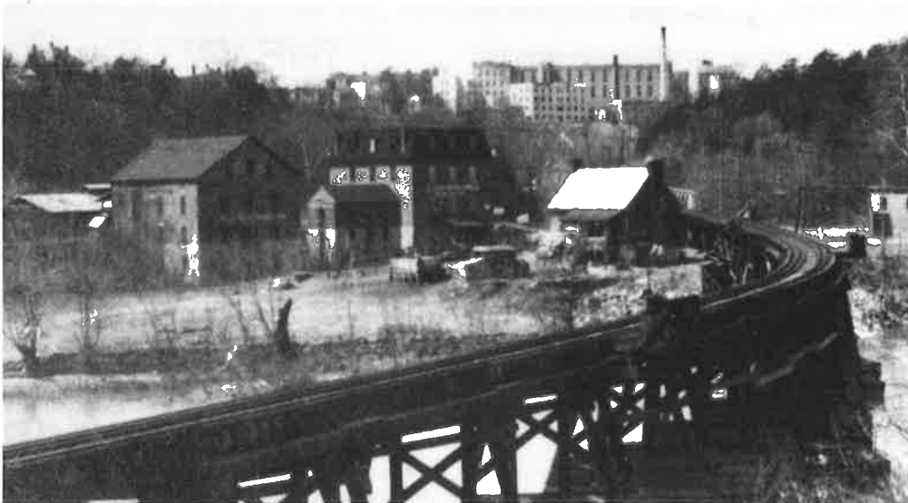
East Lexington, railroad trestle crossing Maury River, 1937
