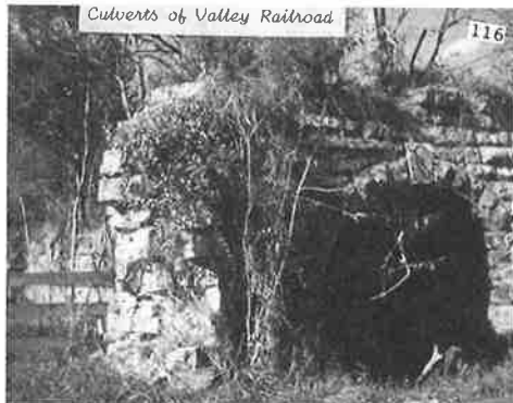
Valley Railroad Culvert on Plank Road
