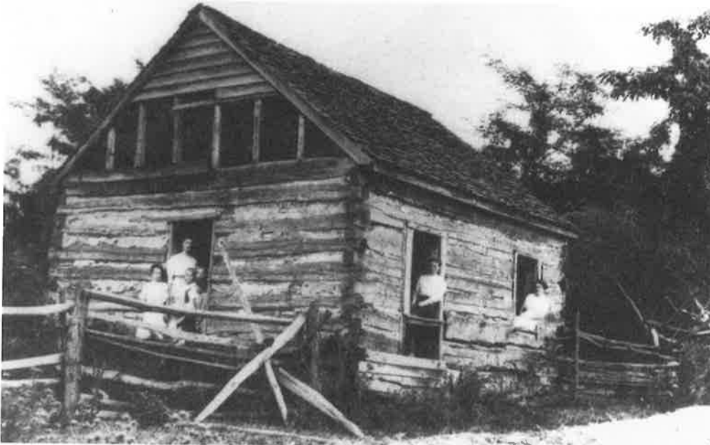
Old School on Timber Ridge
