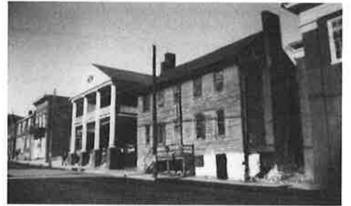
Glasgow House and Jordan House, Main Street, Lexington, Virginia
