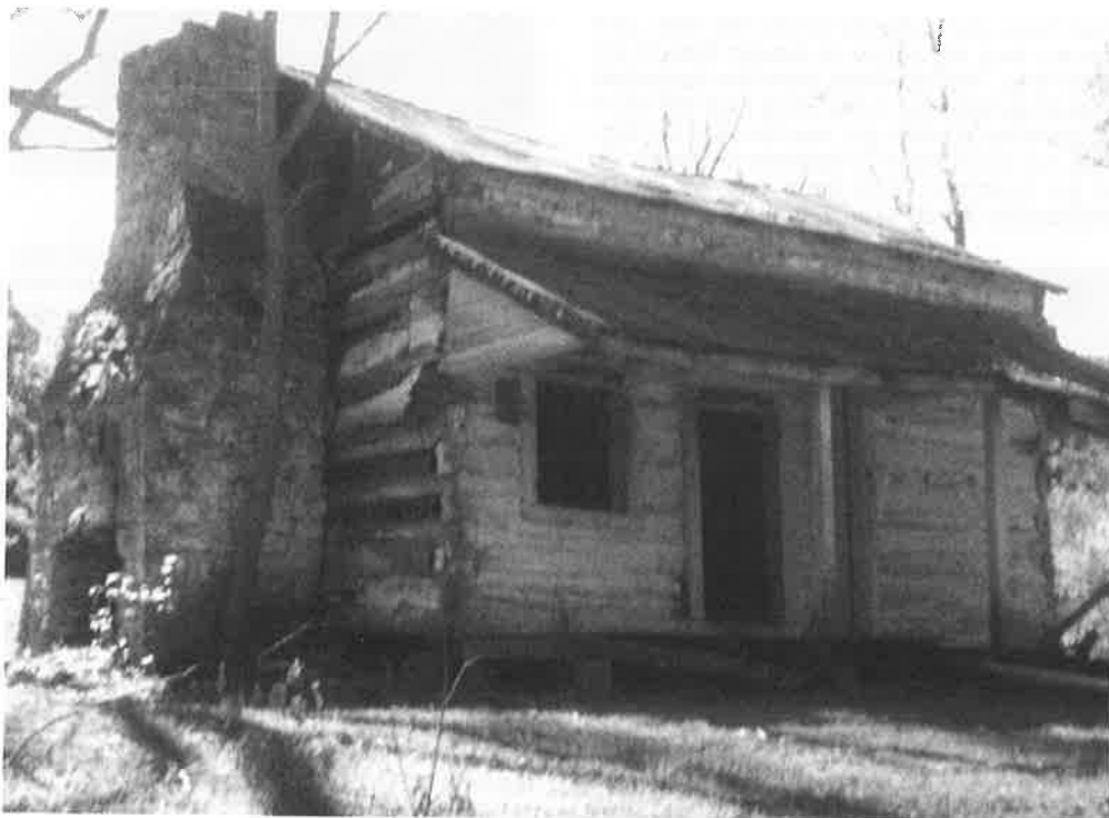
Old Log House
