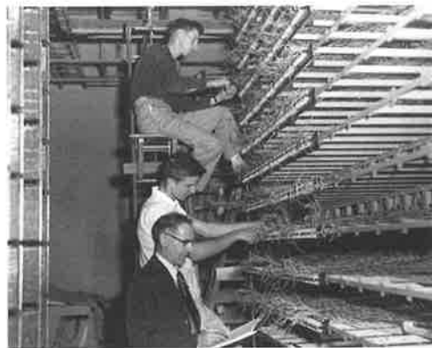
Central Office Repairmen Installing New Frame for Dial Service - 1956. R. L. Rexrode (Top), W. R. Cash, R. E. Buchanan
