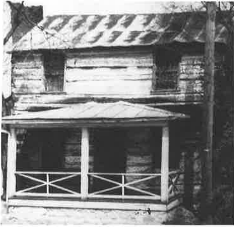
Old Store, Fairfield, Virginia
