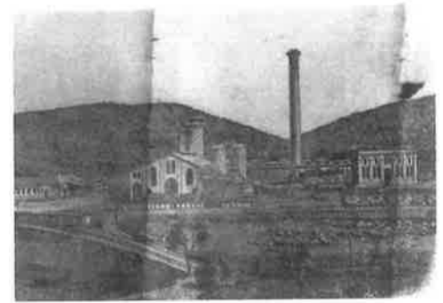
Old Victoria Furnace
