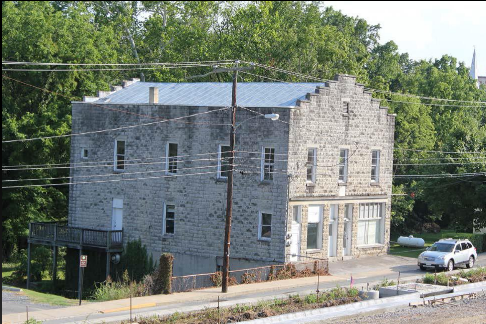
Knights of Pythias Hall -- 1926 Recently wheeled a half-block down Main Street, 2014 (VMI Construction at Bottom, First Baptist Spire, at Right)
